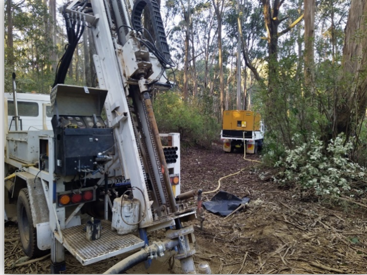
Percussion drilling rig with support truck carrying compressor in the background
